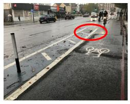
11. GENERAL – The carriageway behind the waterfilled barriers and also cycle track behind the cyclinders appears to be susceptible to the buildup of fallen leaves. Continued build up of leaves and other detruitus may become a slip/skid hazard to cyclists in the track or pedestrians stepping into the widened "footway" areas. Whilst it is recognised that this is largely a maintenance issue, it may require remedial measures to enable regular street sweeping activities to remove the leaves.
