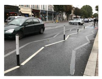
10. The southernmost cylinder north of the Ritherdon Road northbound floating bus stop had been knocked over. It is not clear how it occurred but may require the crossover turning movements to be tracked to check that manoeuvres can be completed without overrunning the cylinder to determine whether to replace or remove it.
