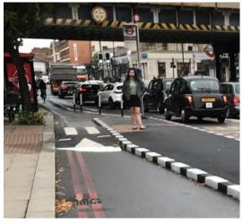
3. Pedestrian refuge island by Elmfield Road – The absence of centerline markings on the northbound approach to the island results in a risk of the corner of the island being struck albeit an illuminated bollard is present.
